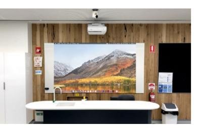
functionality from the touch of a keypad. An Epson Document Camera, and an audio system comprising of a ceiling amplifier, and 4x 8" flush mount ceiling speakers completed the solution. A Crestron TSW-760 touch screen wall mounted media presentation controller was installed to allow users to control the system from the front.
