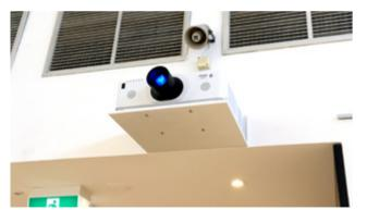
The new Duckboard Function Centre at Austin Health's Repat site in Heidelberg combines both iPad and Crestron control systems, emphasising the integration of all aspects of the audio visual spectrum. A high brightness Hitachi projector was installed on a custom wall bracket - projecting onto a fixed frame screen - while Audac column speakers, a subwoofer and a custom lectern completed the solution.
